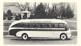
"The Flexible Clipper," ultra-streamlined bus, carries 20 passengers, and is powered by 78 h. p. engine. With safety glass throughout, de luxe chairs and down pillows are provided.
