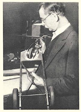
A third wheel shown in model is designed to remove weight from towing car and to end rear spring and axle breakdown. Device eases riding by removing much swaying and bobbing.
