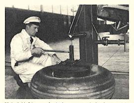
United Air Lines mechanic demonstrates device developed for quick and easy removal of tires from air liners. Jack and auto rim device loosens and forces tire from airplane wheel.
