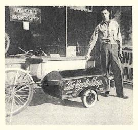
Designed for camping or delivery use, this midget bicycle trailer built by William Moll, of Minneapolis, Minn., has a built-in radio controlled from the bicycle's handlebars.
