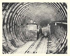
This Diesel powered locomotive is used to haul heavy loads in a tunnel 95 feet below the streets of London, England. Exhaust fumes are removed from tunnel by a filter device.
